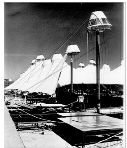
Partially-completed tensile membrane roof.
